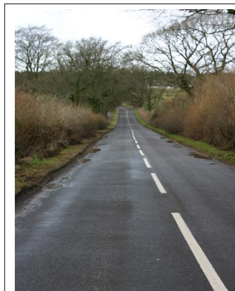
Broken road edges and tyre tracks. Just how deep are the puddles?
